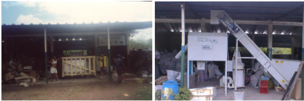
Picture 5.8: Installation and operation of the glass mill
